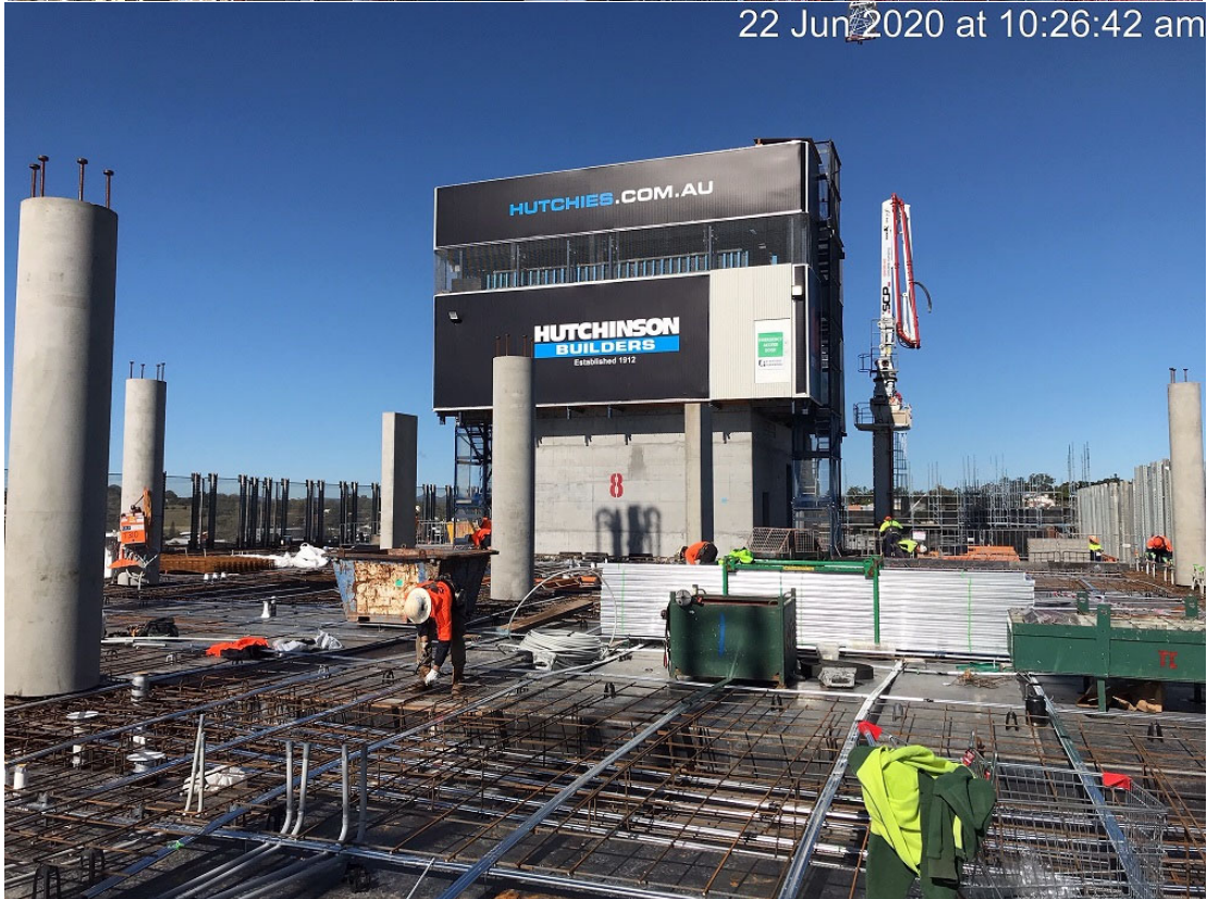
Administration Building: Level 08 slab reinforcement.
