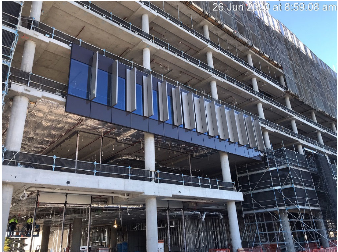
Administration Building: Curtain wall installation commencing.
