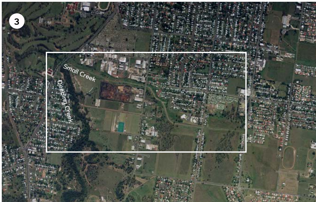
Small Creek, Raceview in 2002. Concrete swale within mown grassed area. (Source: QImagery)
