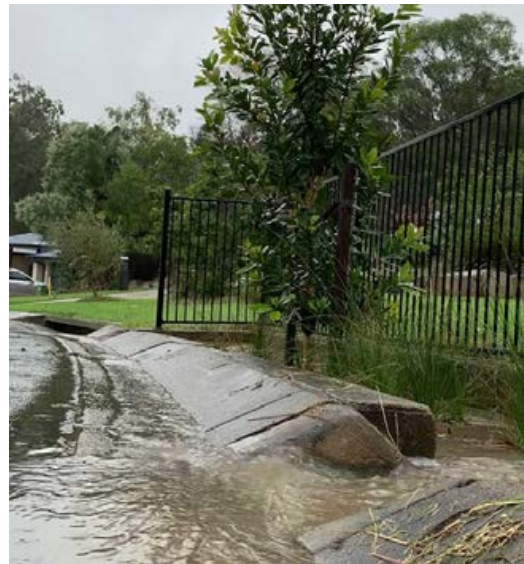
Same tree and sedges irrigated by stormwater run-off in May 2022.
