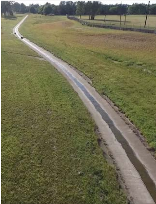
Small Creek Pre 2016 – Concrete swale within a maintained grass drainage corridor. (Source: Ipswich City Council)
