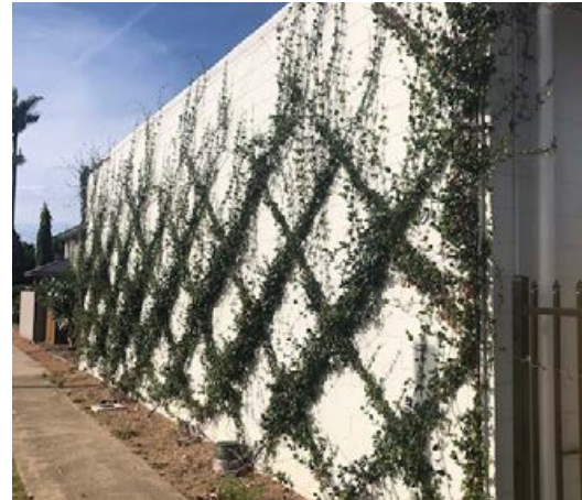
Greening treatment to building wall in Townsville. Stainless steel trellis with climber.
