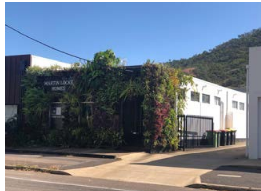
Green wall to single story building in Townsville.
