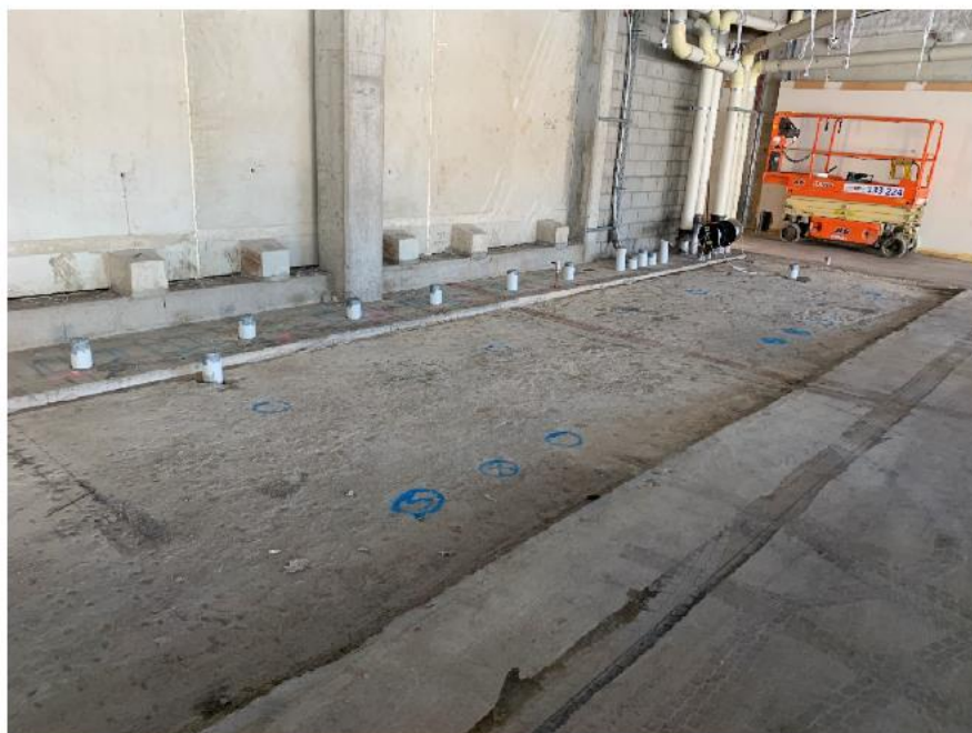
Under-slab drainage installed to Lv1 amenities
