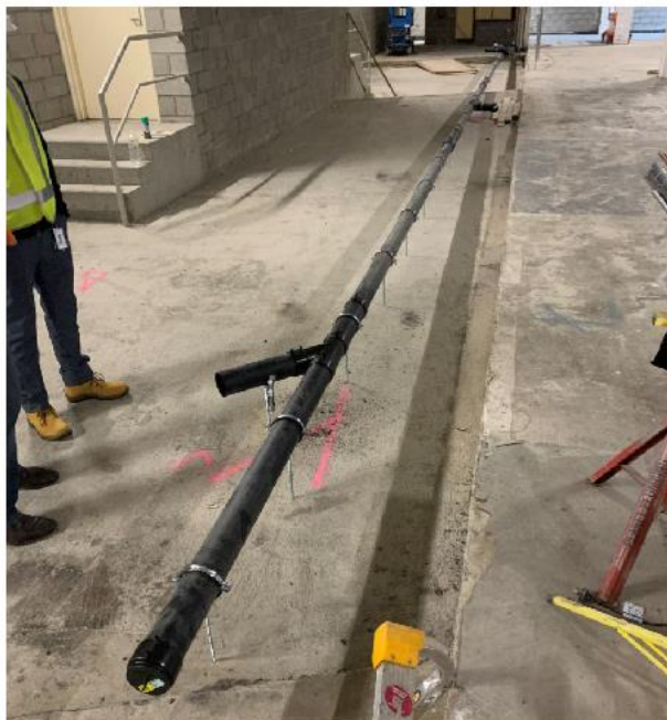
Installation of in-ground drainage to Ground Floor tenancies.
