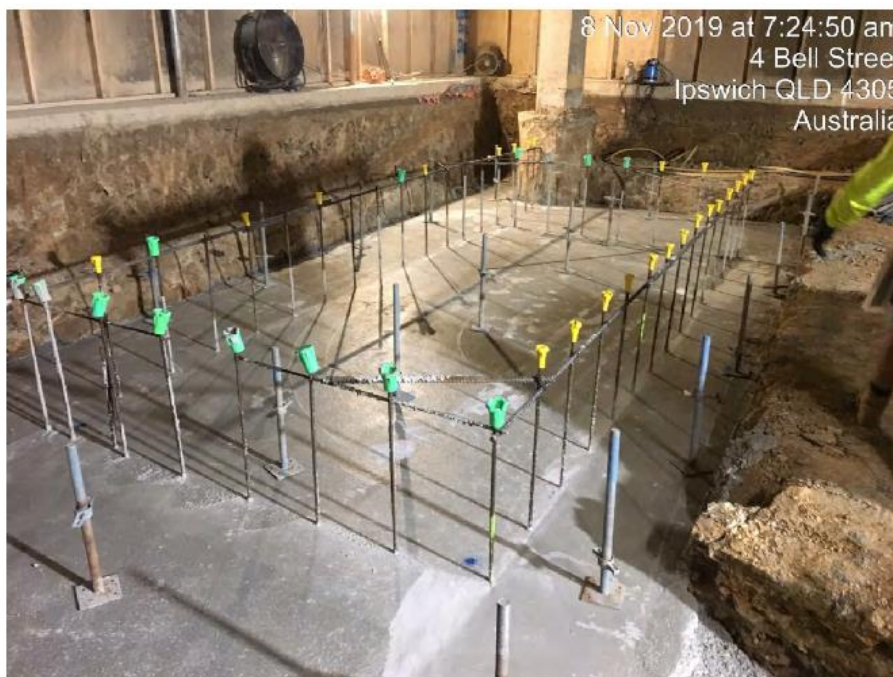
Civic Carpark: Concrete footings poured to lifts 3 & 4 at Basement
