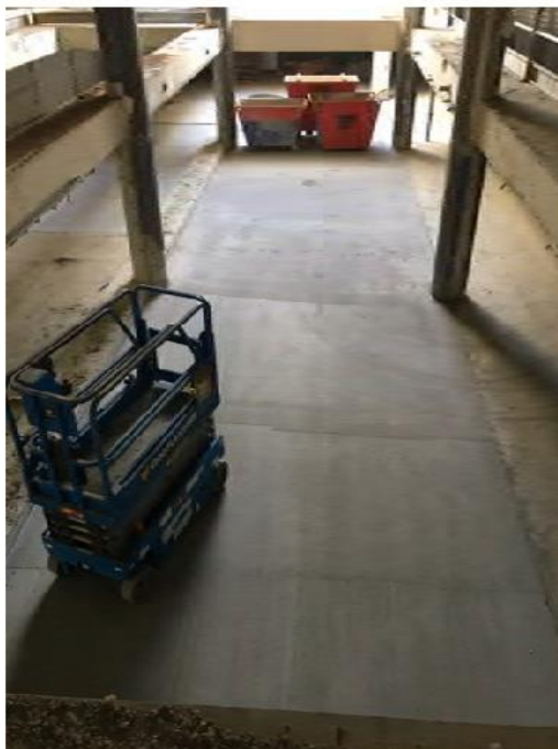
Civic Carpark: Concrete slab infill for the opening of the removed travelator
