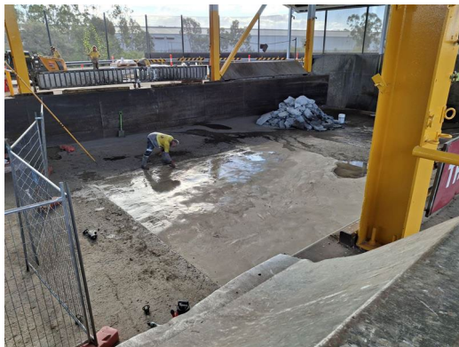
Completing the surface.
