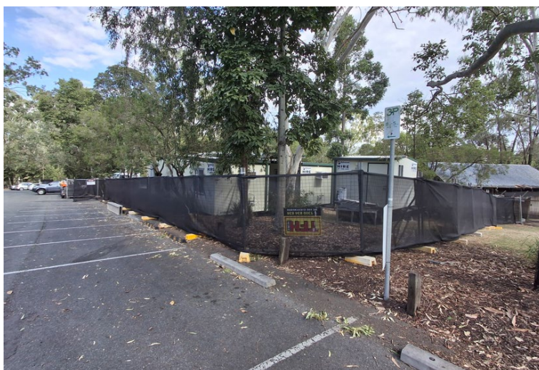
Temporary staff facilities.
