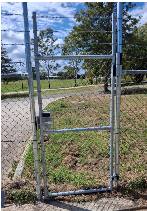
New pedestrian access gate installed.
