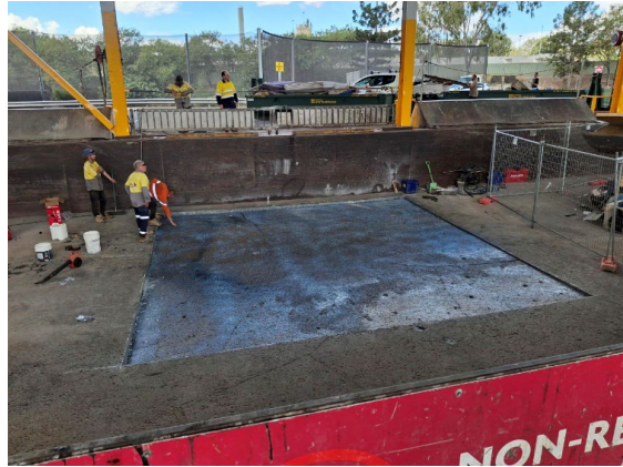
Applying the adhesive to a clean, excavated surface.
