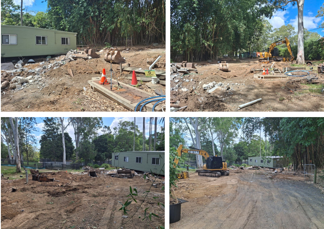
Demolition of the existing facilities.
