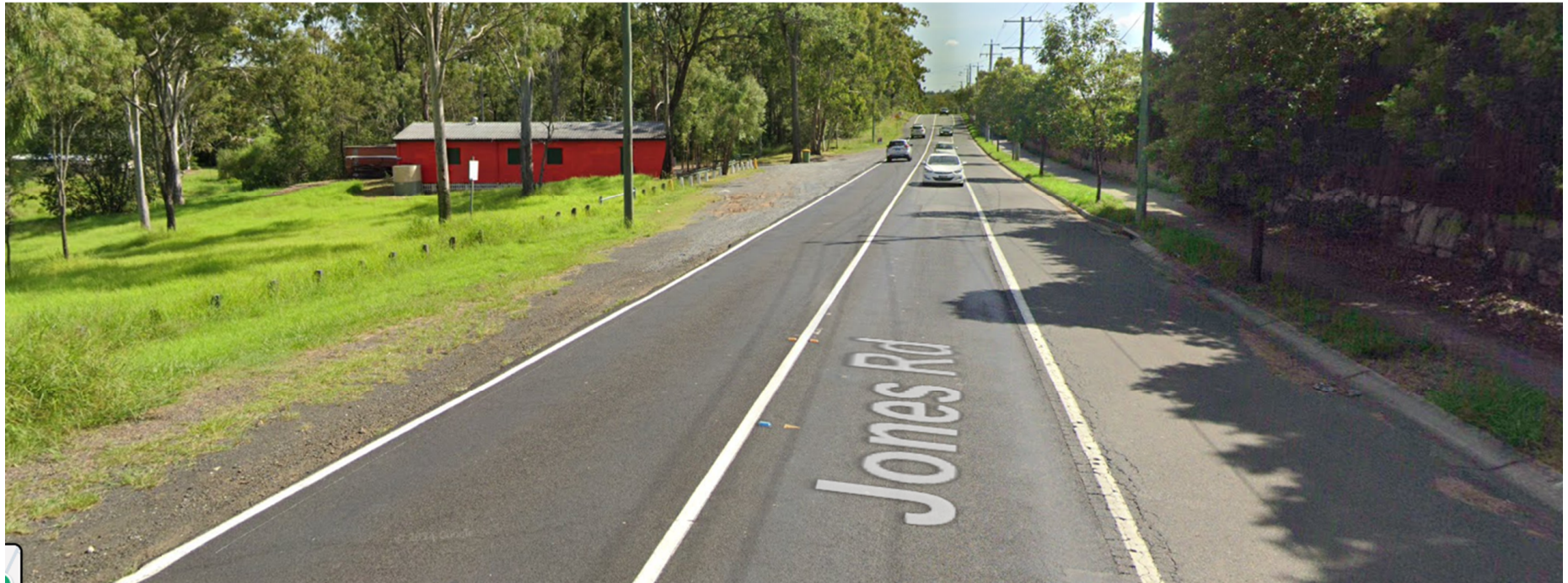
Image northbound near Redbank Plains Scout Den
