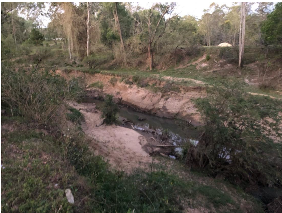
Figure 4 WO002 Woogaroo Creek bank erosion after floods and Celtis removal.
