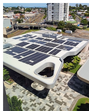
Pictured: Completed installation.
