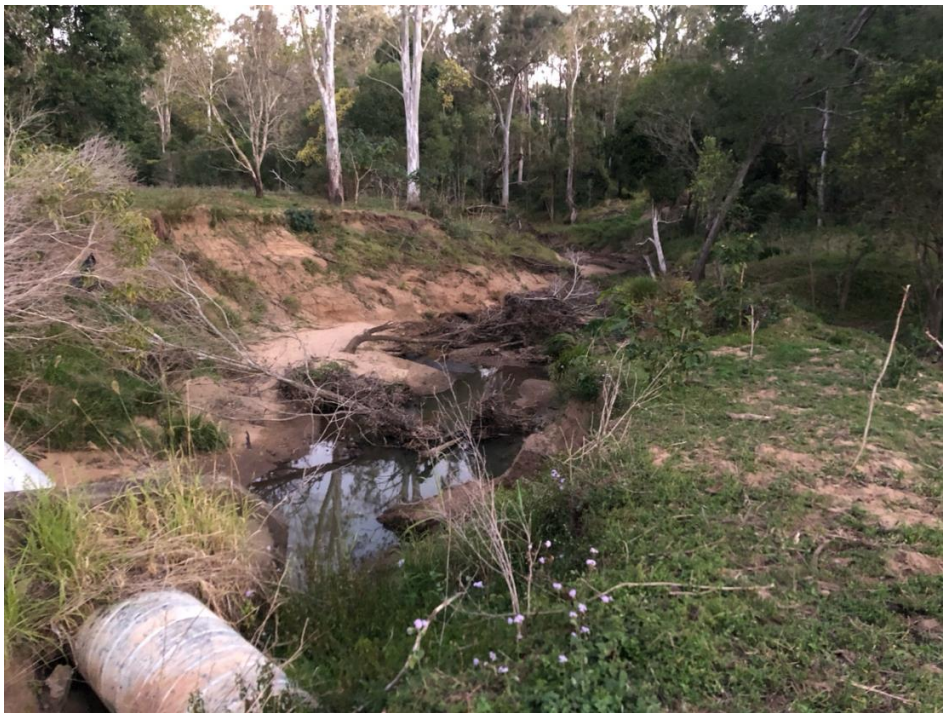
Figure 3 WO002 Woogaroo Creek bank erosion after floods and Celtis removal.
