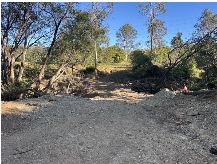
Figure 6 WO002 Landholder constructed bridge over creek creating a barrier.
