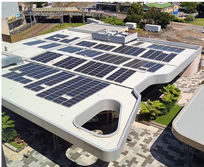
Pictured: Nicholas St Library 200kW system.
