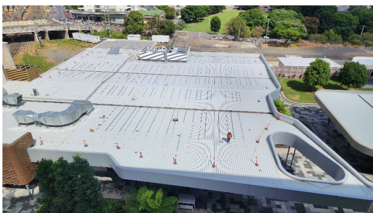
Pictured: Installation has commenced.
