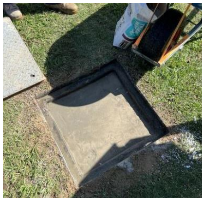
Figure 2 - Redland City Council - Cable pit filled with sand
