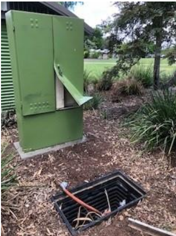
Figure 3 - Ipswich City Council - Electrical cable theft damage
