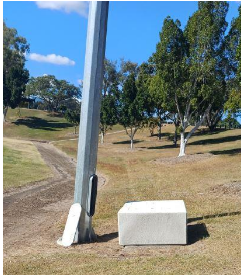
Figure 5 - Concrete block on top of cable pit
