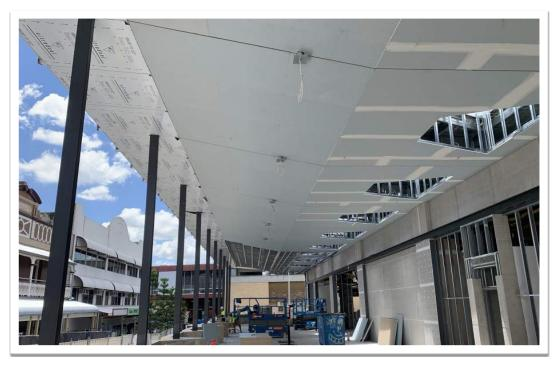
Soffit being sheeted to awning over Union Place dining area.
