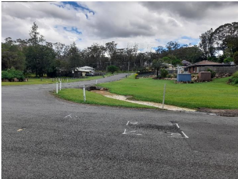
View South from Frontage towards short St and drainage path.
