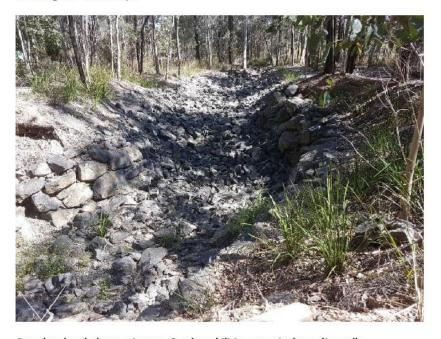
Completed rock chute at Ironpot Creek, stabilising an actively eroding gully.
