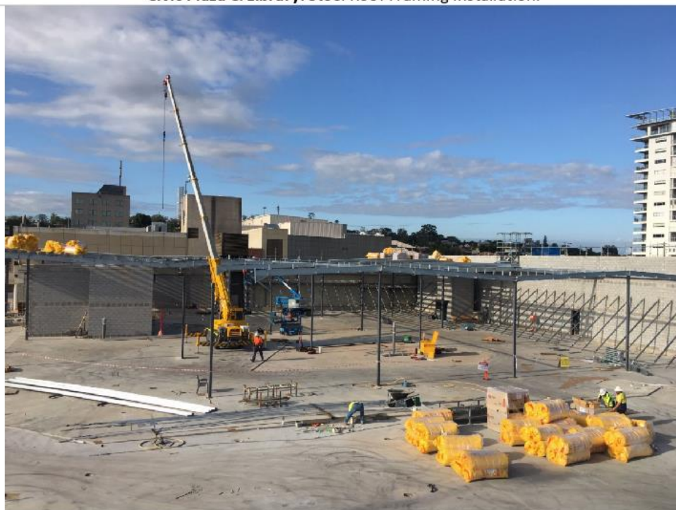
Civic Plaza & Library: Steel Roof Framing Installation.
